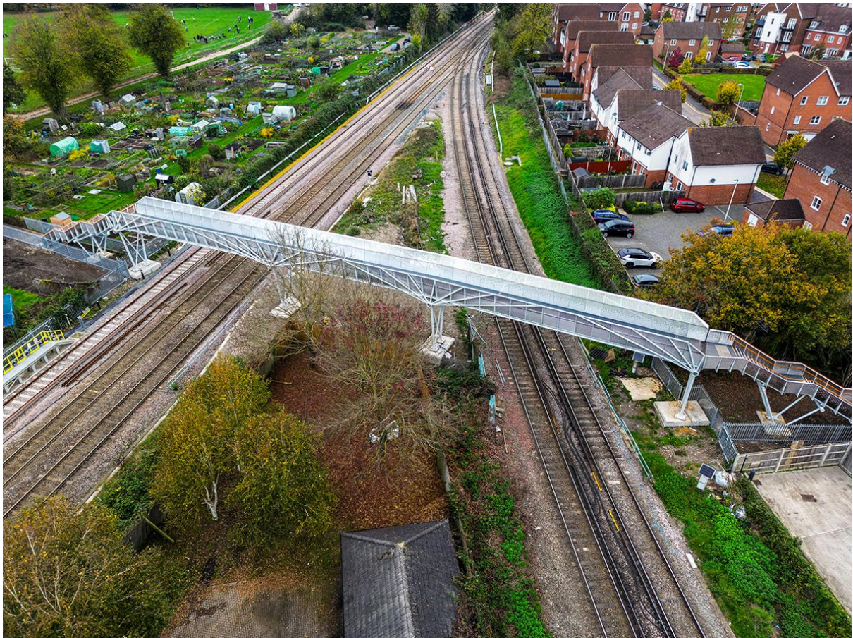
Figure 6. Satellite view of the bridge installed
