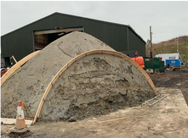
Figure 6. Completed clay mould
