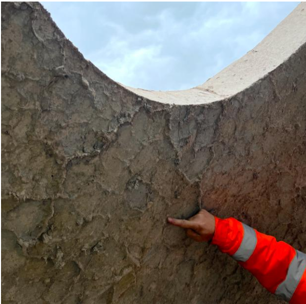
Figure 12. Cracking of the concrete
